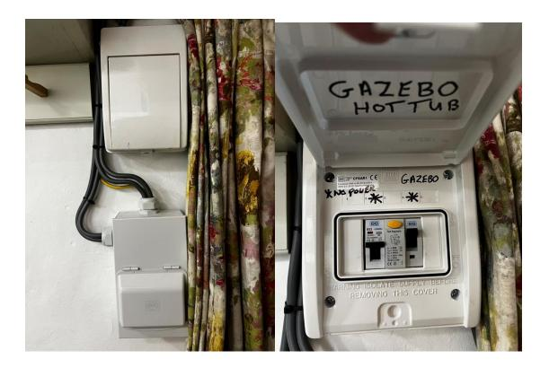
6. The lower box has the switch to swap power from the mains supply to our generator. The switches are normally in the UP position which means mains power is selected. So, once the generator is running, move them DOWN to select generator power. Push the switches down- they might be stiff. Once you do this, lights and power will be restored in the house.
